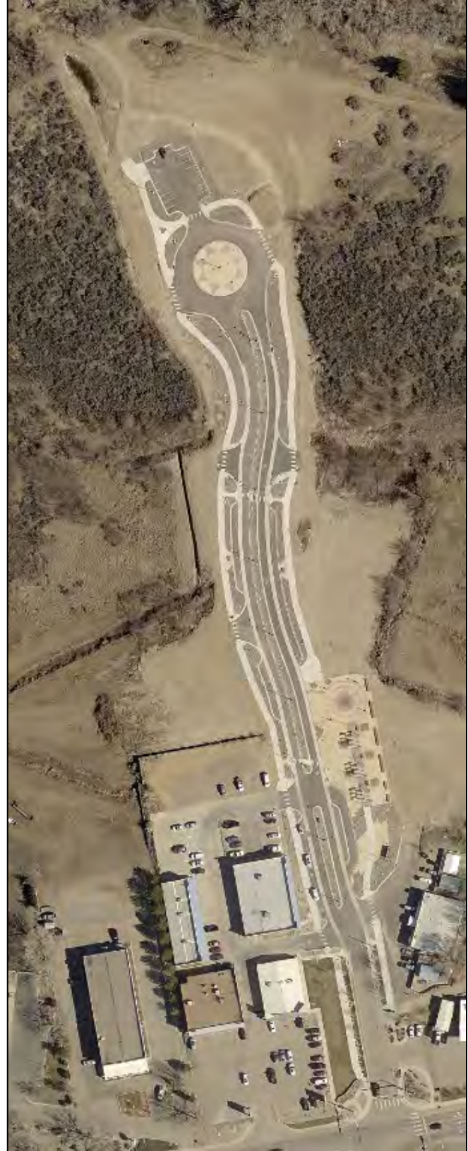
Figure 4.4. North Main Extension.
