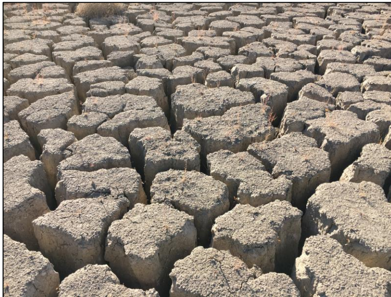
Figure 2 – Cracking in the surface of the pond adjacent to Boring No. B-2.
