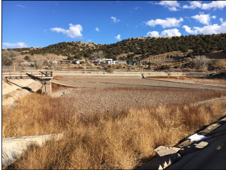
Figure 1 – View looking east from the top of the embankment from the northwest corner of the pond.
