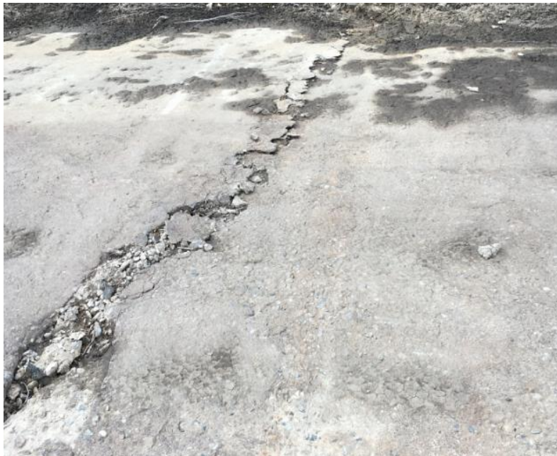
Figure 10 – Longitudinal Crack with Delamination
