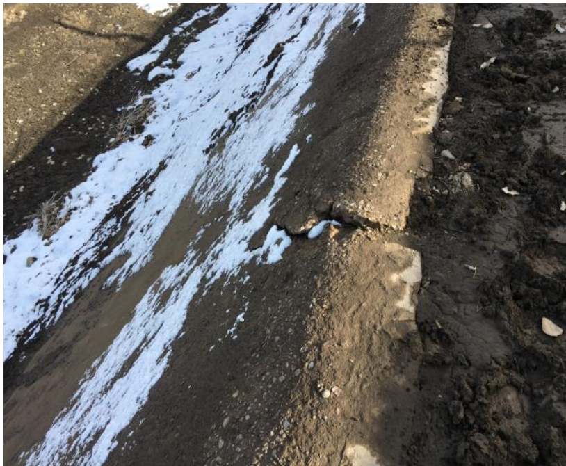
Figure 14 – Longitudinal Crack
