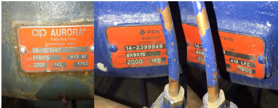
Figure 25 – Pump Nameplates
