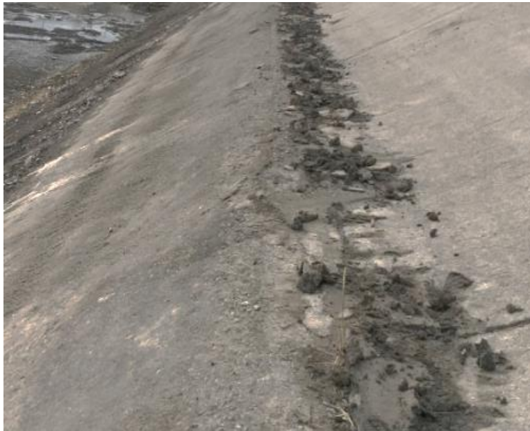
Figure 7 – Signs of Spalling
