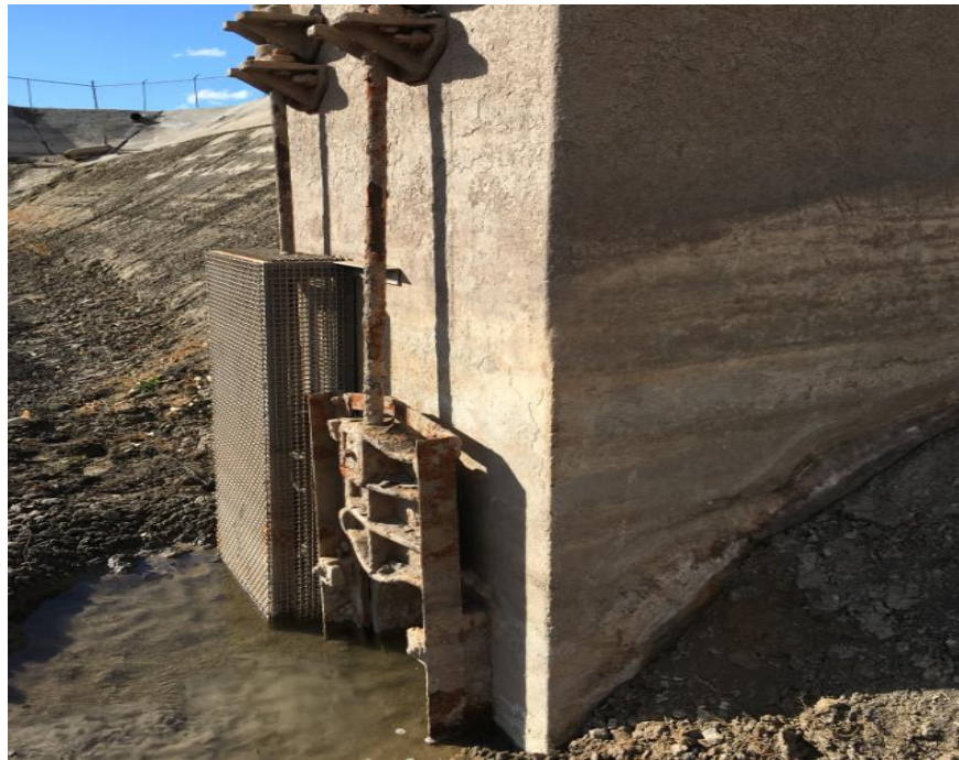
Figure 19 – Leaching at lower right corner of figure
