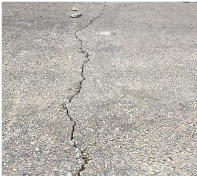
Figure 8 – Longitudinal Crack
