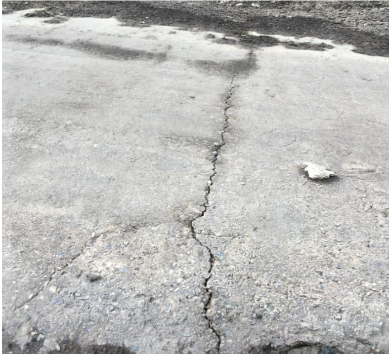
Figure 9 – Longitudinal Crack
