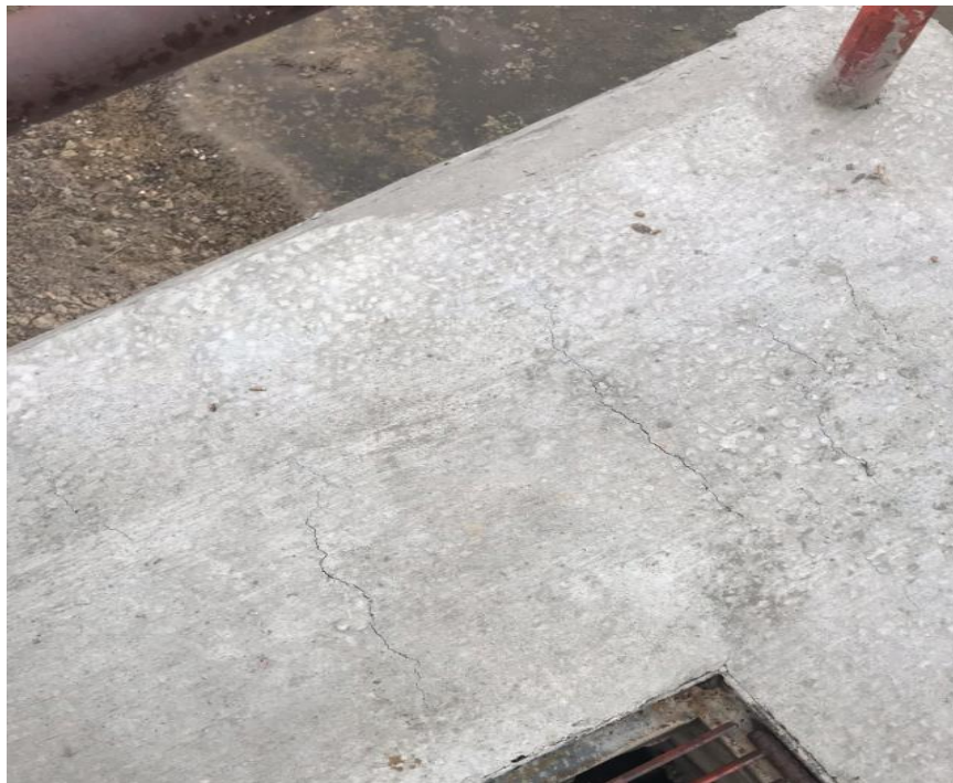
Figure 22 – Nominal Cracking
