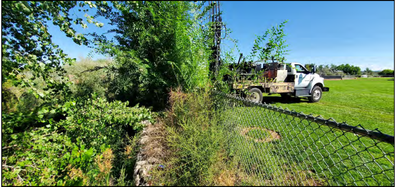
Drill Rig at Boring B-2 View Towards the North
