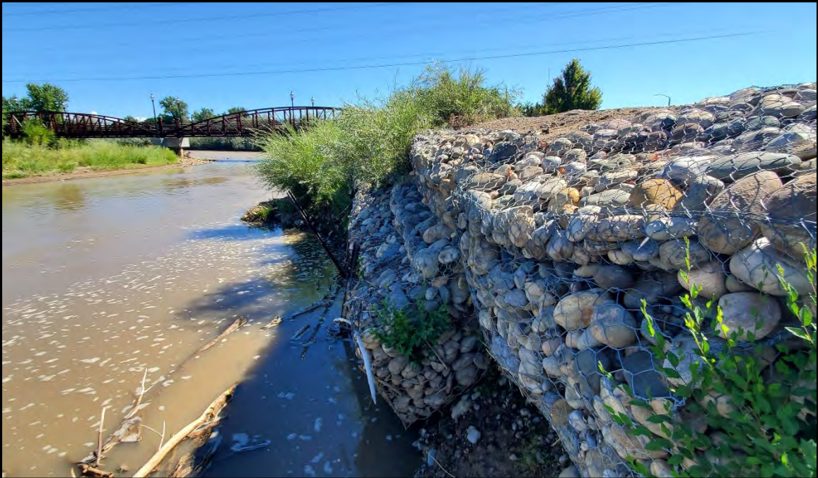
Riverview of Gabion Wall near Boring B-4 View Towards the East
