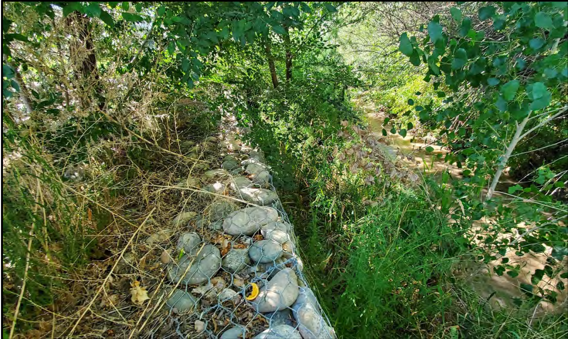
Gabion Wall near at Boring B-2 View Towards the South
