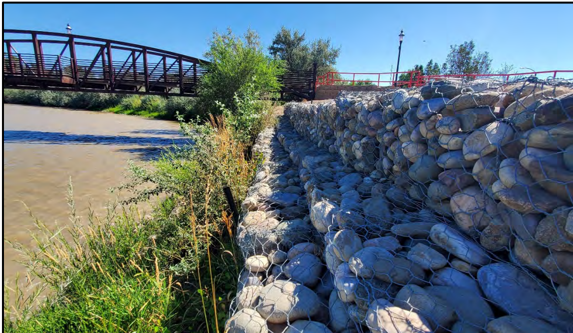
Riverview of Gabion Wall near Boring B-5 View Towards the East
