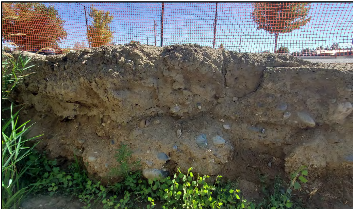
Fill Behind Gabion Wall near Boring B-3 View Towards the East
