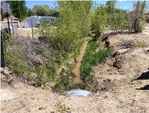
Figure 1. Culvert and drainage near Blanco Street and Creekside Village, looking southeast, 2023.
