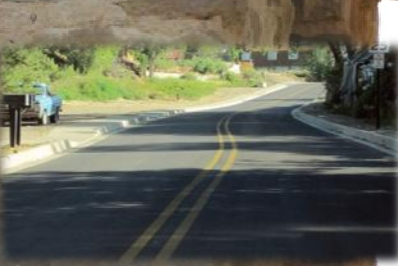
Oliver Drive Improvements
