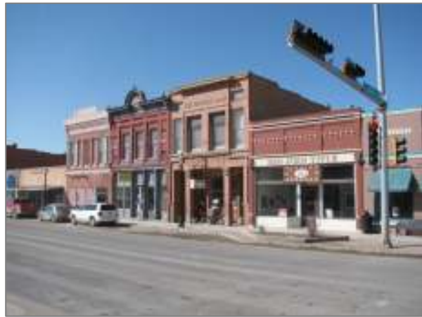
Main Avenue revitalization elements include sidewalk improvements and streetlights
