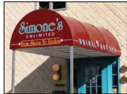
Example of attached canopy.
